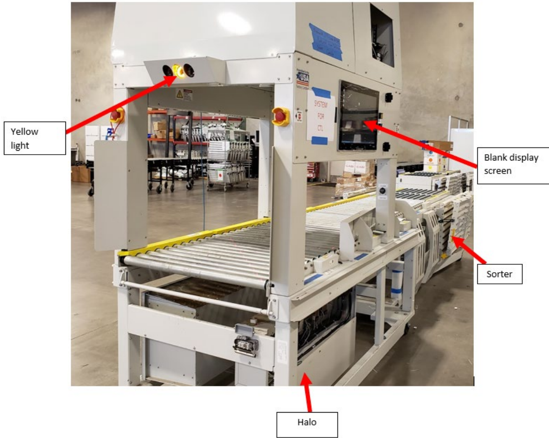
Figure 2 - Halo Scanner Connected to Tee Sorter
