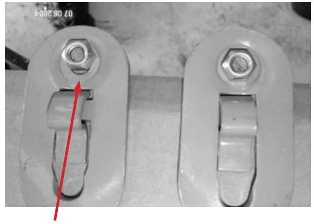
Notice space under the nut this hook is seriously worn and must be replaced immediately.
