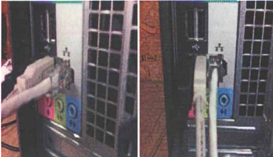
Figure 7. Installing Network Cable
