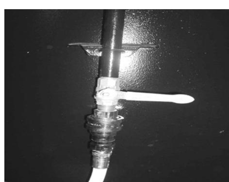
**14. With your insulated gloves on, close the ball valve and disconnect the hose from the tank**
