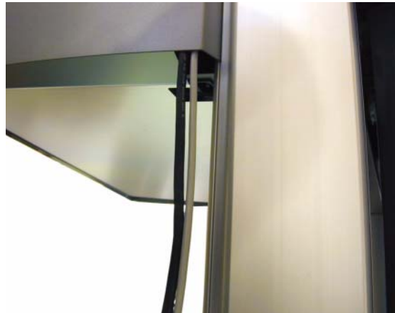
Figure 20: The cables run inside the left side plate.
